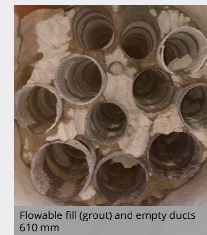
Steel pipe 1200 mm with empty pipes made of plastic and steel embedded in insulating material
