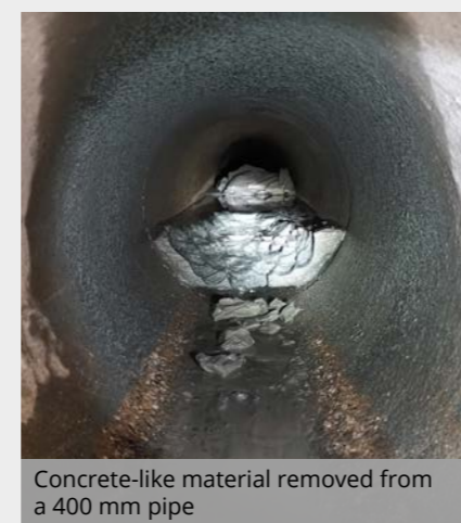
Concrete suspension in PVC pipe 400 mm
