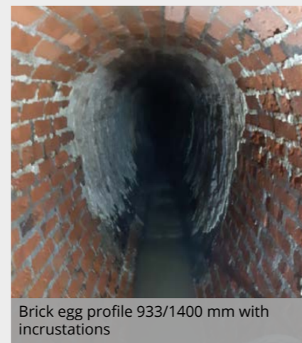
Dissolved lime with growth layers
